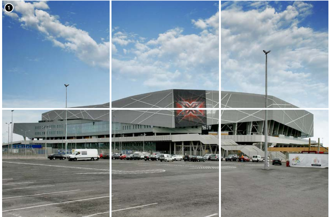
1. Lviv Stadium – Lviv, Ukraine. built for the purposes of the EURO 2012 Football Championships, equipped in a modern sprinkler installation consisting of the KAN-therm Sprinkler System
